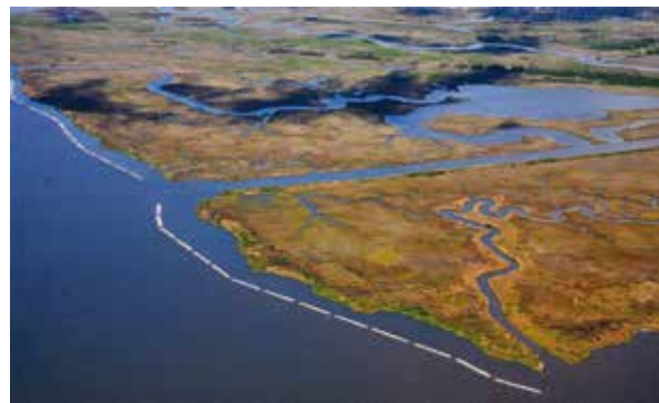
FIGURE 9 Hancock County Marsh living shoreline project, Mississippi living shoreline sills (Photo credit: Ramseur, 2020).
