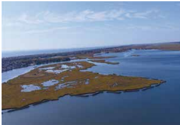
FIGURE 8 Shooting Island, New Jersey living shoreline sills (Photo credit: Anchor QEA and ACT Engineers).
